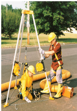
Manhole Tripod Setup
