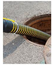
Calif. Greenbook 2021 Section 3-12.5.2 Sewage Bypass and Pumping Plan. ...Bypass pump suction and discharge lines that extend into manholes shall be rigid hose or hard pipe. Lay-flat hose will not be allowed to extend into manholes...
